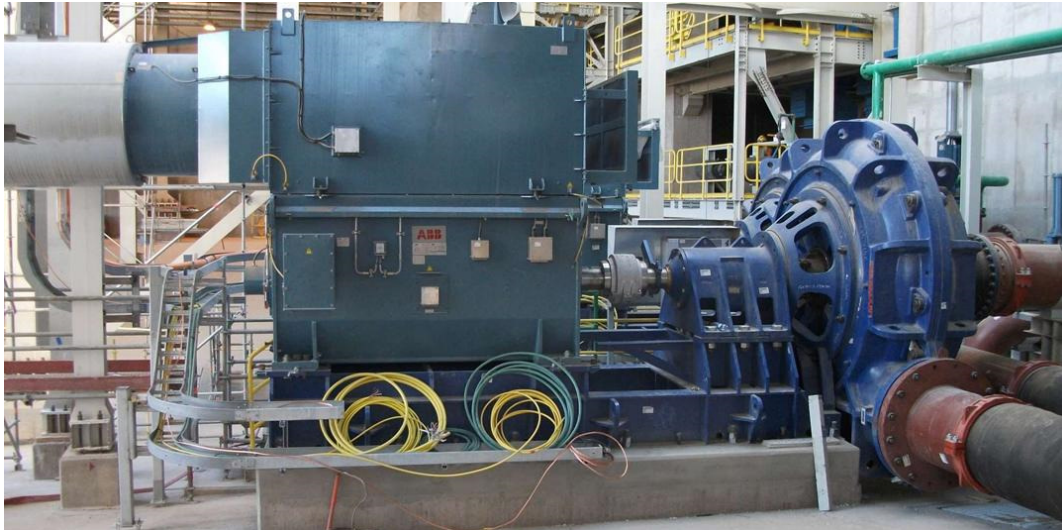
Figure 13 – Discharge positions, Position “G” – Warman® MCR® 650 pump
