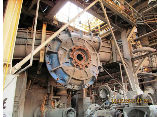
Figure 53 – Wet End Disassembly for Warman® Pump
