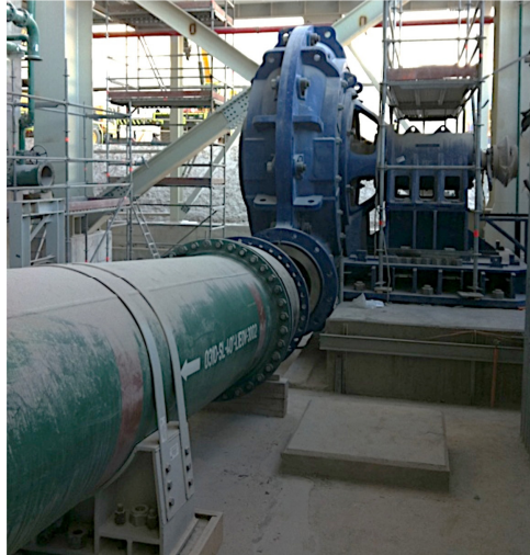
Figure 10 – Discharge positions, Position “G” – Warman® MCR® 650 pump
