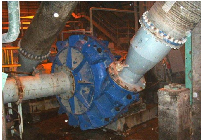
Figure 20 – Warman® MCR® 450 pump, Discharge Position “K”.
