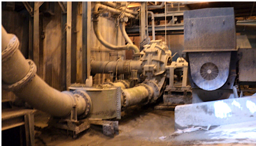
Figure 11 – Discharge positions, Position “G” – Warman® AH® 20x18 pump
