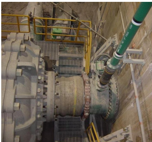
Figure 26 – Expansion Joint, 900 mm Inner Diameter
