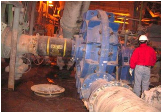
Figure 22 – Warman® MCR® 450 pump, Suction modification.
