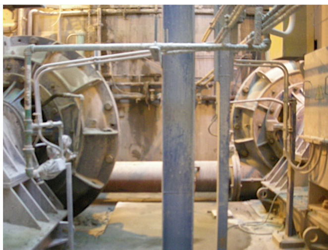
Figure 12 – Discharge positions, Position “G” – Warman® MCR® 550 pump
