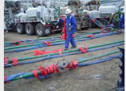
SPM technician on site installing FSR
